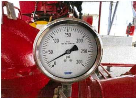
Discharge pressure gauge
