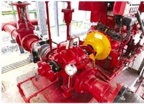
As show Fire pump condition
