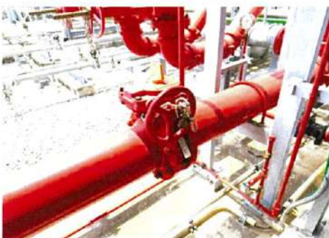
Test pipeline control valve
