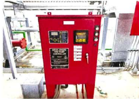
Fire pump controller
