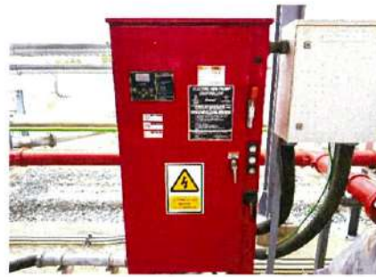
Fire pump controller
