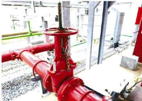
Suction isolate valve opened
